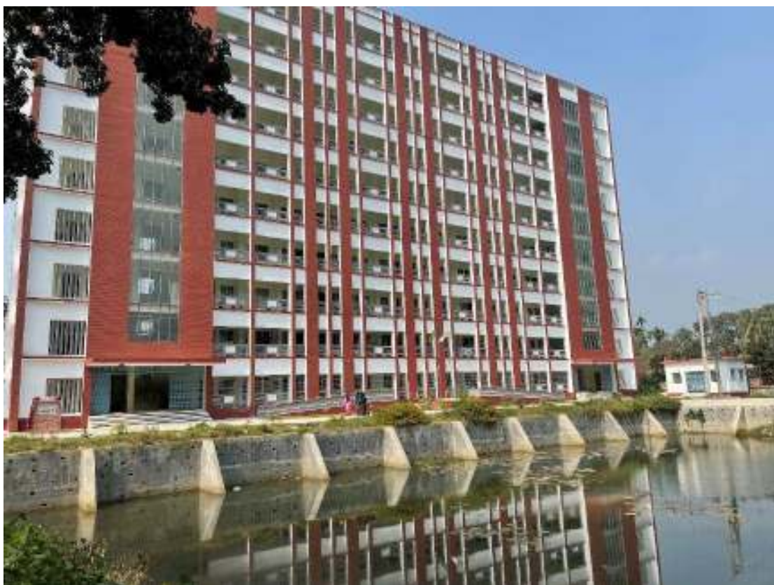
Photo 13: Newly built 10-storeyed Academic Building
